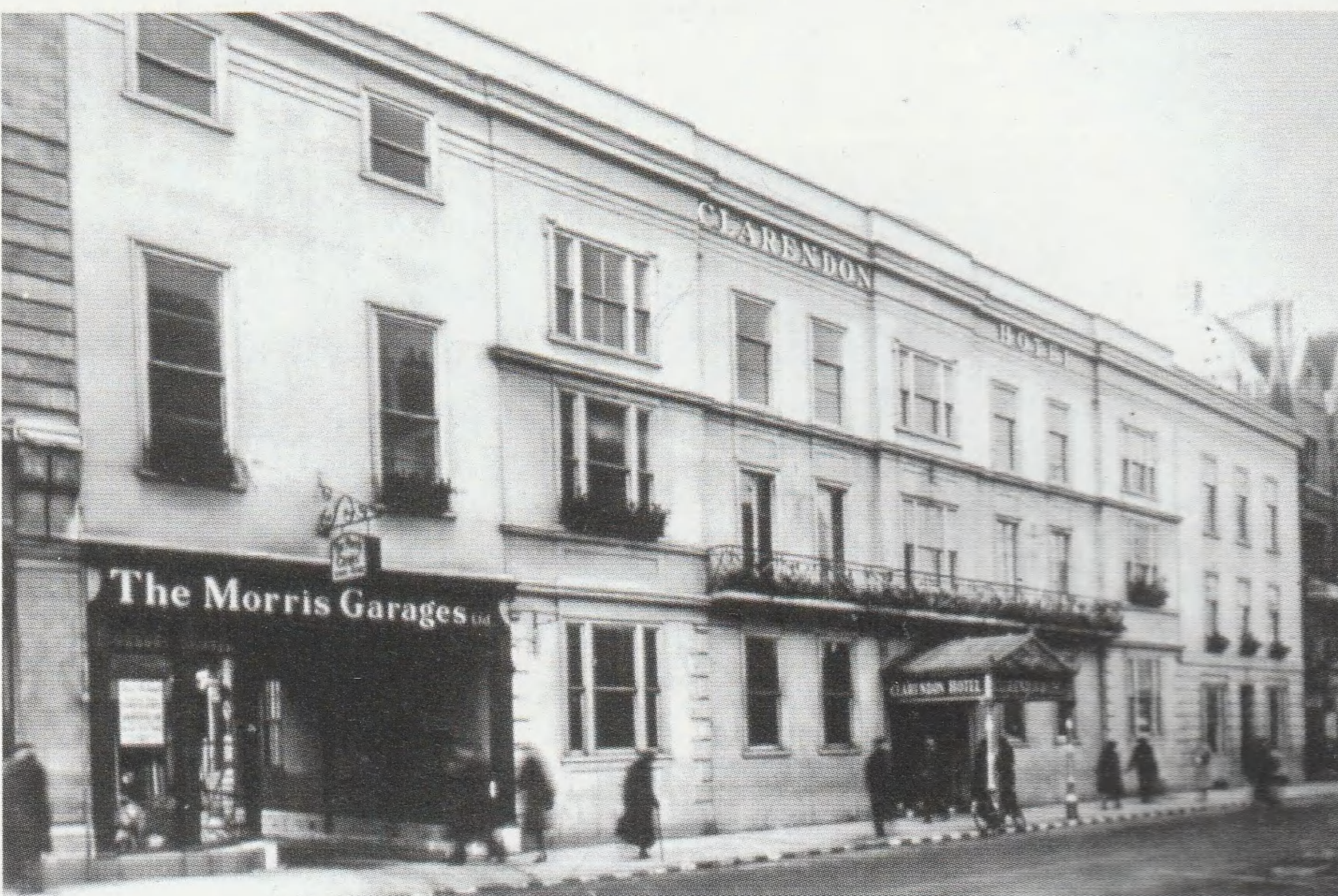
The entrance to the workshops in Cornmarket Street
